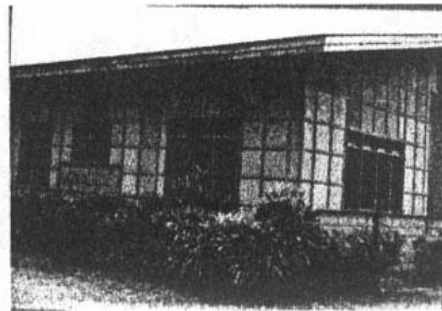
Fig. 10. Workshop building using CWCB as outside walling.
